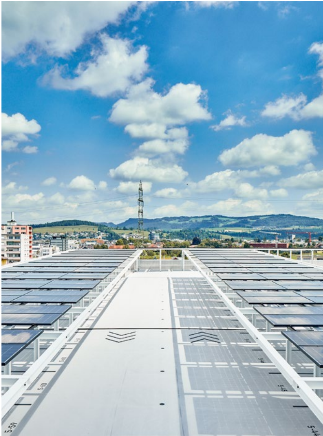
Solar system with an installed capacity of 72.5 kWp at the Mobility Hub in Zug North
